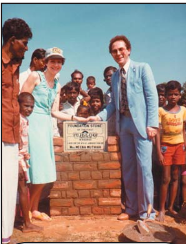
January 8, 1981 : Jo & Brian Millar laying foundation stone of the 1st «Day-Care Centre» Miblou.
